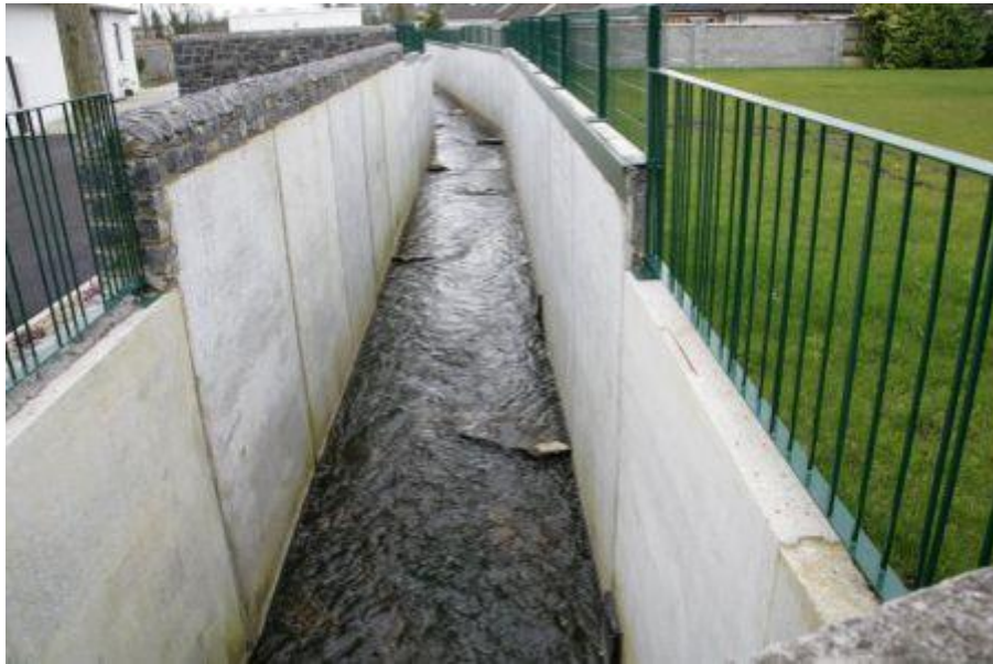
Tullamore River Flood Defences
