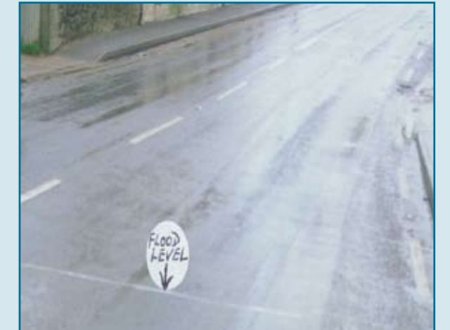
Flood extents marked on a road
