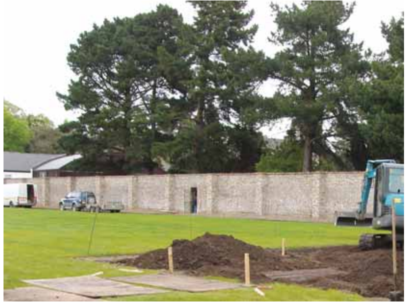
The Garden Under Construction
