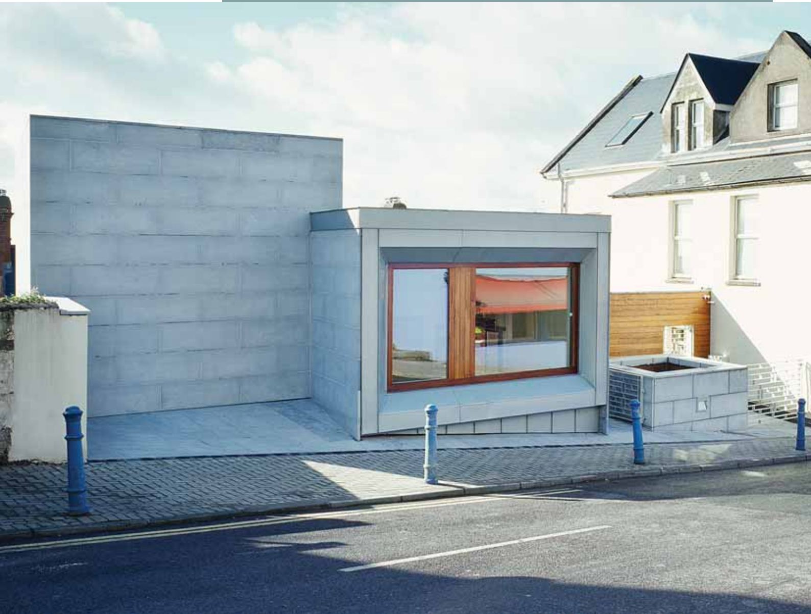
Cobh Custom House, East Beach Road Entrance
