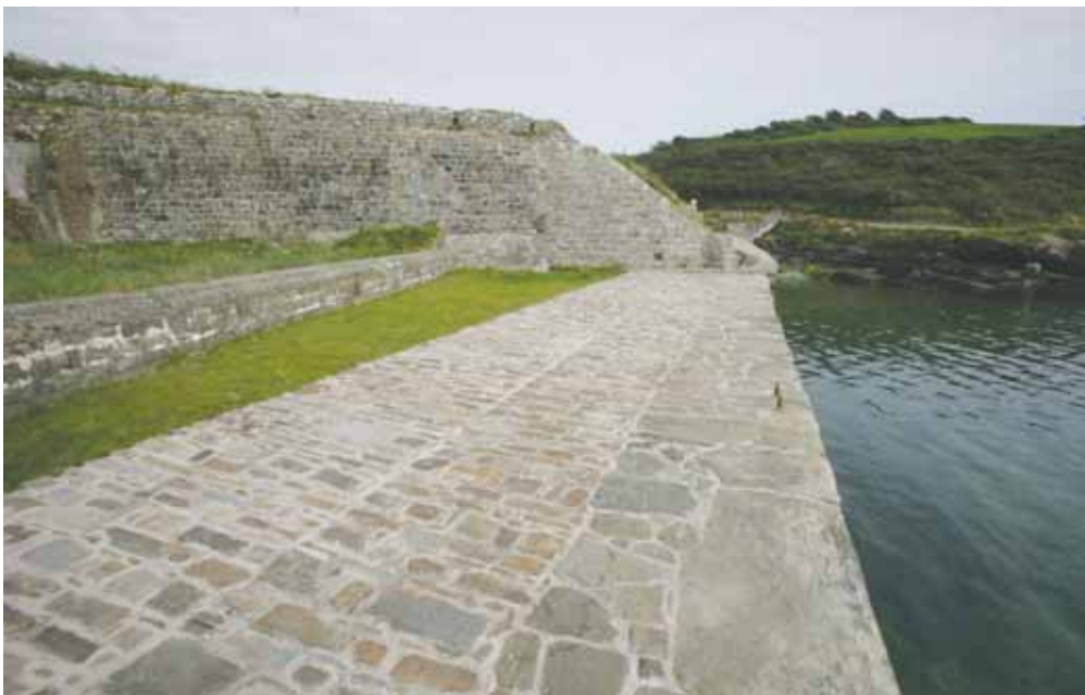
New sandstone surface to quay
