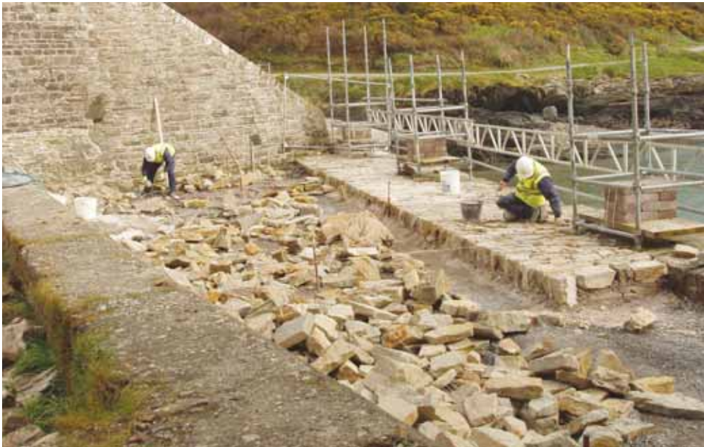
Workforce laying new sandstone surface to quay
