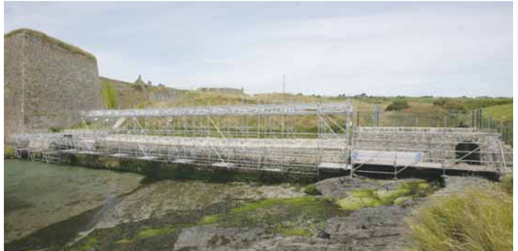
57.0 meters of cantilevered scaffold
